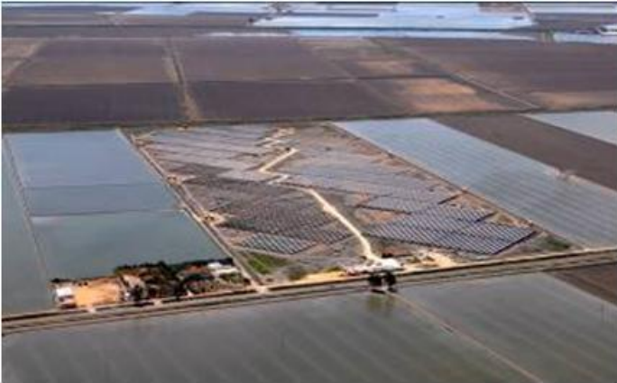
Isla Mayor Spain, 8.4 MW SunPower T0 Tracker
