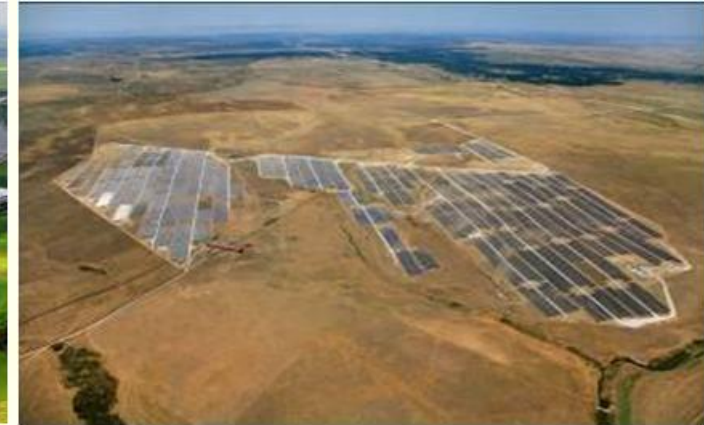
Trujillo, Extremadura, Spain-Elecnor 23 MW SunPower T0 Tracker
