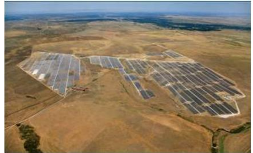
Trujillo, Extremadura, Spain-Elecnor 23 MW SunPower T0 Tracker
